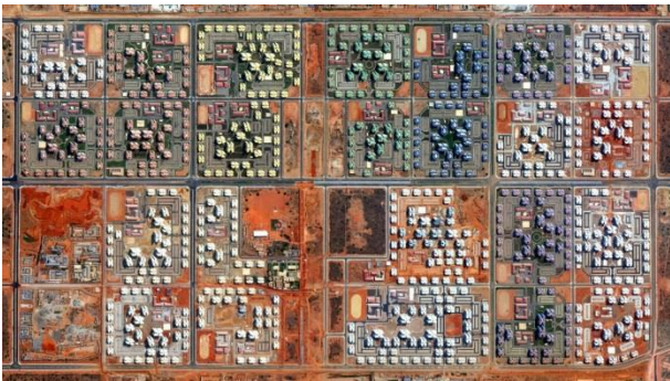
Figure 4. Aerial view of Kilamba
