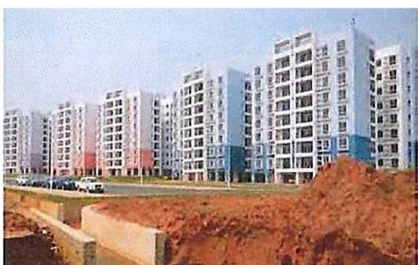
Figure 2. Dundo at street level
